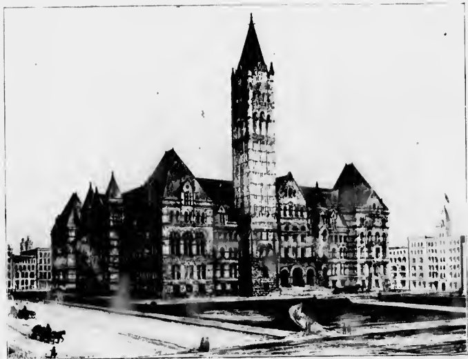
NEW CITY HALL AND COURT HOUSE, TORONTO.
